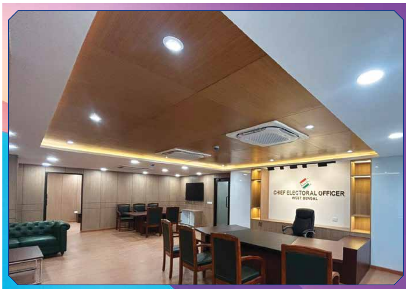
Interior Fitout Works, Office of the Chief Electoral Officer, Govt. of West Bengal
