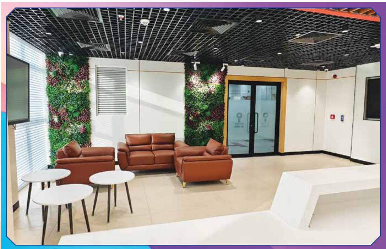
Interior Fitout Work in the office space of Oil India Ltd. at NBCC Square, Kolkata
