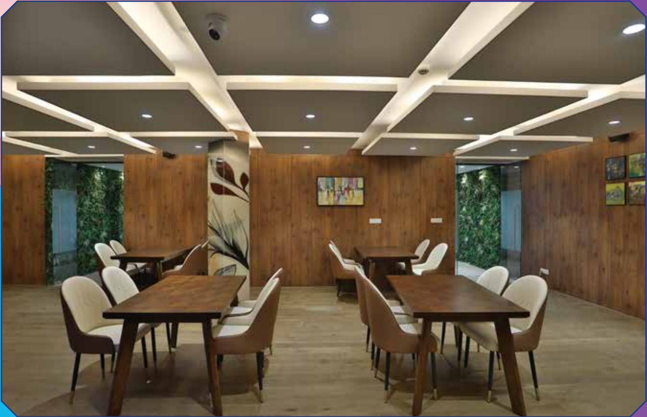
Interior Furnishing & Fit-out work of New ISA Building of IPO Dwarka, New Delhi
