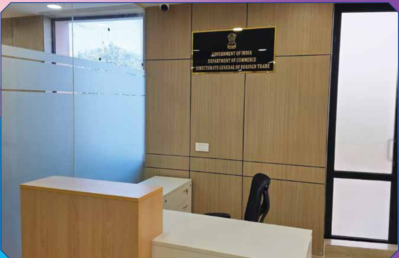
Execution of Interior Fit-out Works at the office of Directorate General of Foreign Trade, New Delhi
