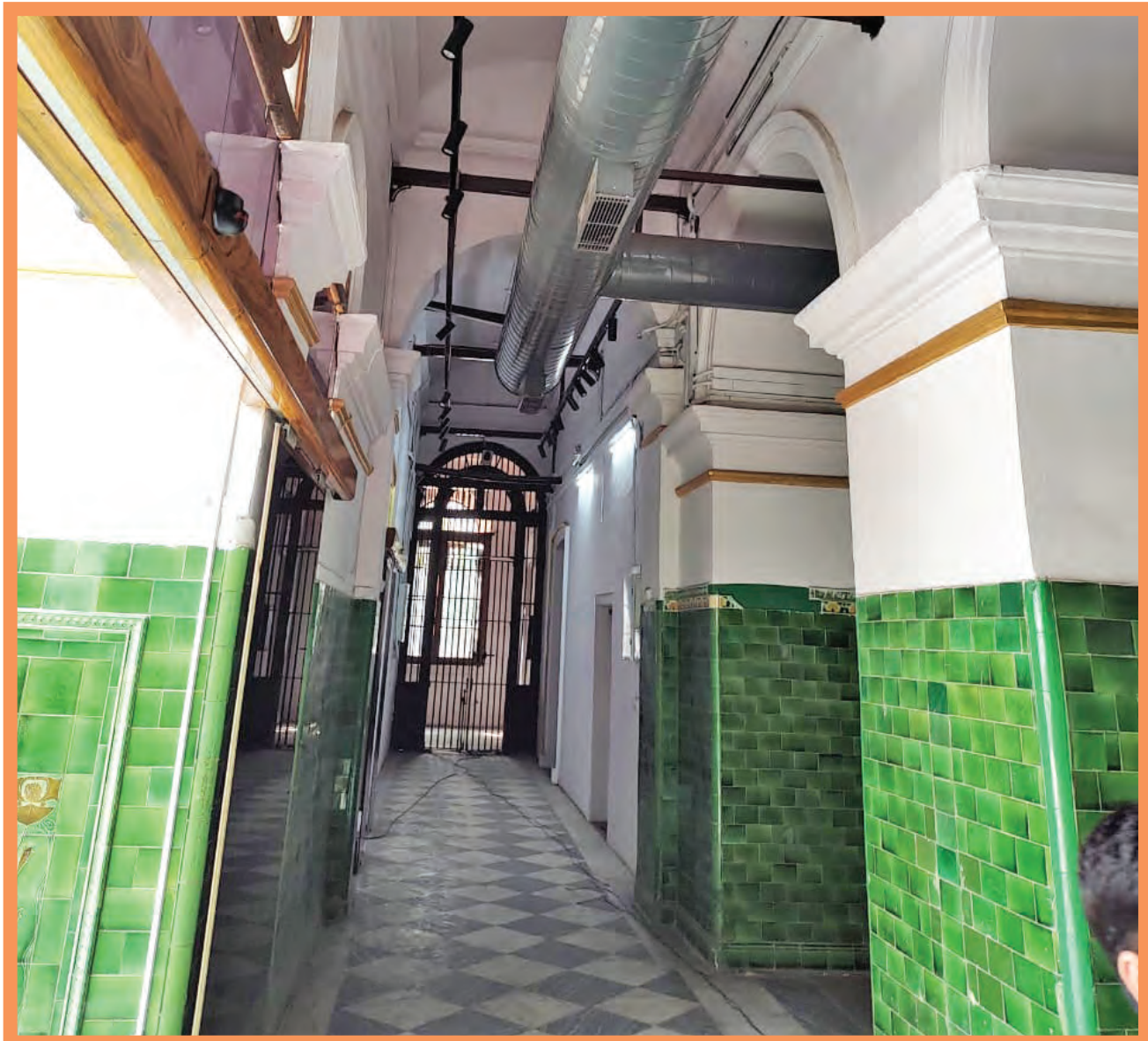
Interior/ Renovations work at National Gallery of Modern Arts, Kolkata
