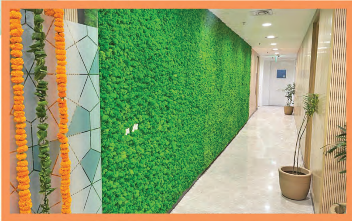
Interior Fit out work at Indian Renewable Energy Development Agency Limited, New Delhi
